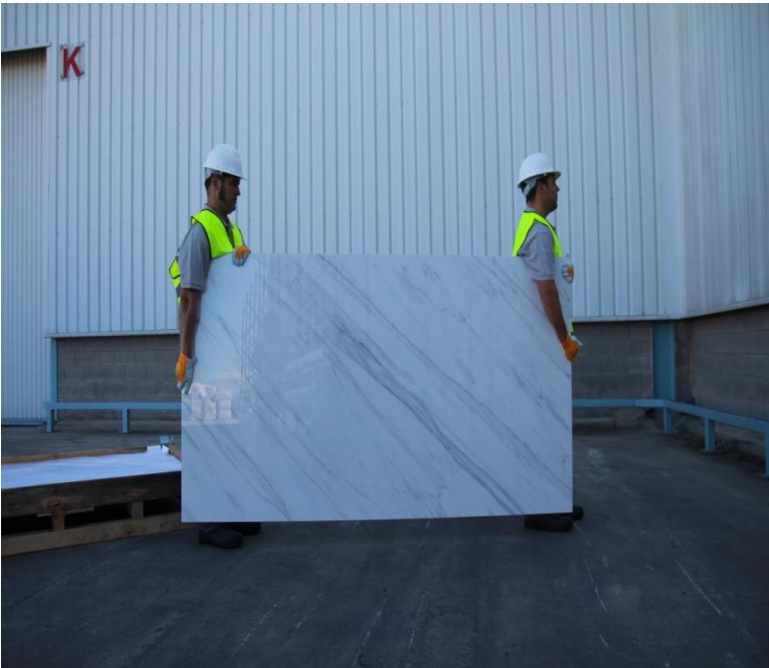
When moving the sheet it is very important to keep it in horizontal position all the time. Keeping the upright position, sheet should be hold on the top part and with both hands.
